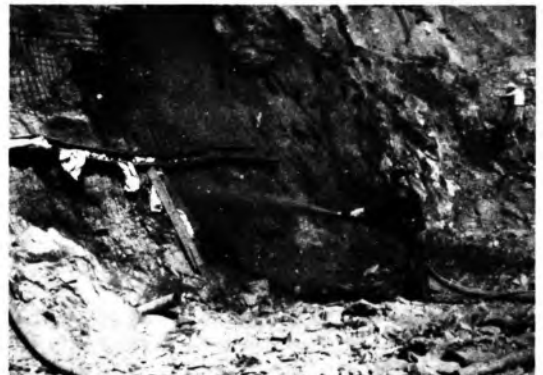
Mapping of excavated surfaces before shotcrete is important in construction phase
